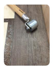
Install the next plank adjacent to the first plank, overlap the interlocking tab ensuring edges are aligned. Make sure seams are tight without any size (large or small) gaps. If necessary, use a straight edge, level or equivalent to ensure back edges are aligned. Use a hand roller or non-marking rubber mallet to firmly secure the end seams. End seams should be level and flush when secured and not overly compressed.
