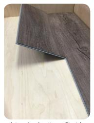
or pre-determined pattern. Start by holding the plank at a slight angle while interlocking the length of the planks together. Once completely engaged lower the plank flat ensuring there are no gaps.
