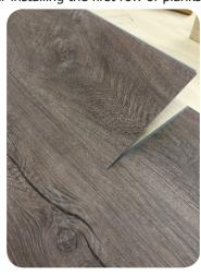
align and interlock length of next by lightly butting corner of first plank. Do not over compress to first plank. Drop into place and hand roll all seams for a tight and level fit. Proceed with rest of installation. End cuts from one row at finishing wall can be used to start next
